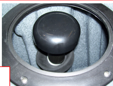
Float Shutoff Assembly
